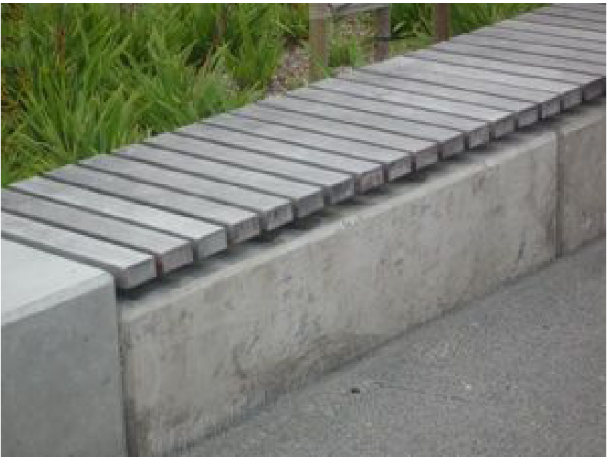
CONCRETE BENCH WITH WOOD SLAT SEAT TOP
